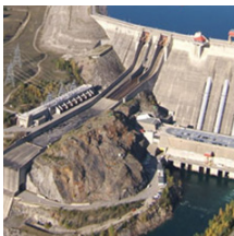
BC Hydro proceeding with work on Revelstoke 6
