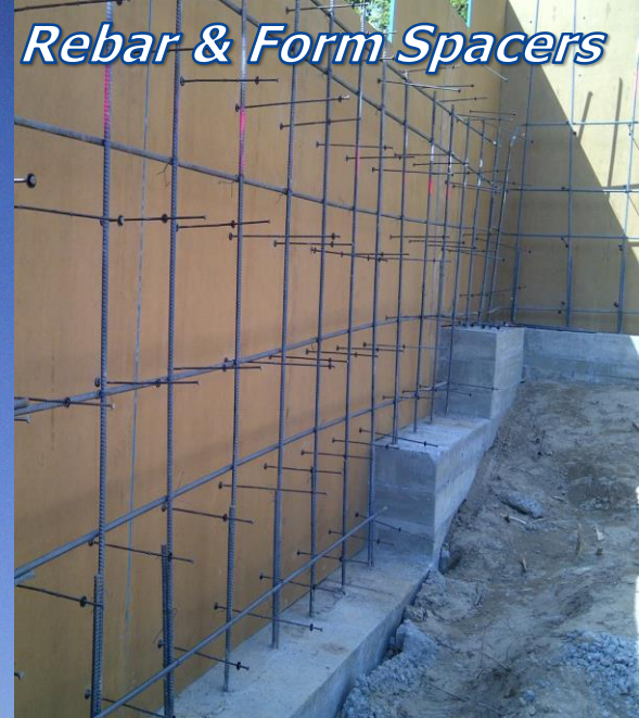
Forming Foundation & Retaining Wall
