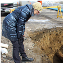
Rossland public works repairs damaged pipes on Spokane
